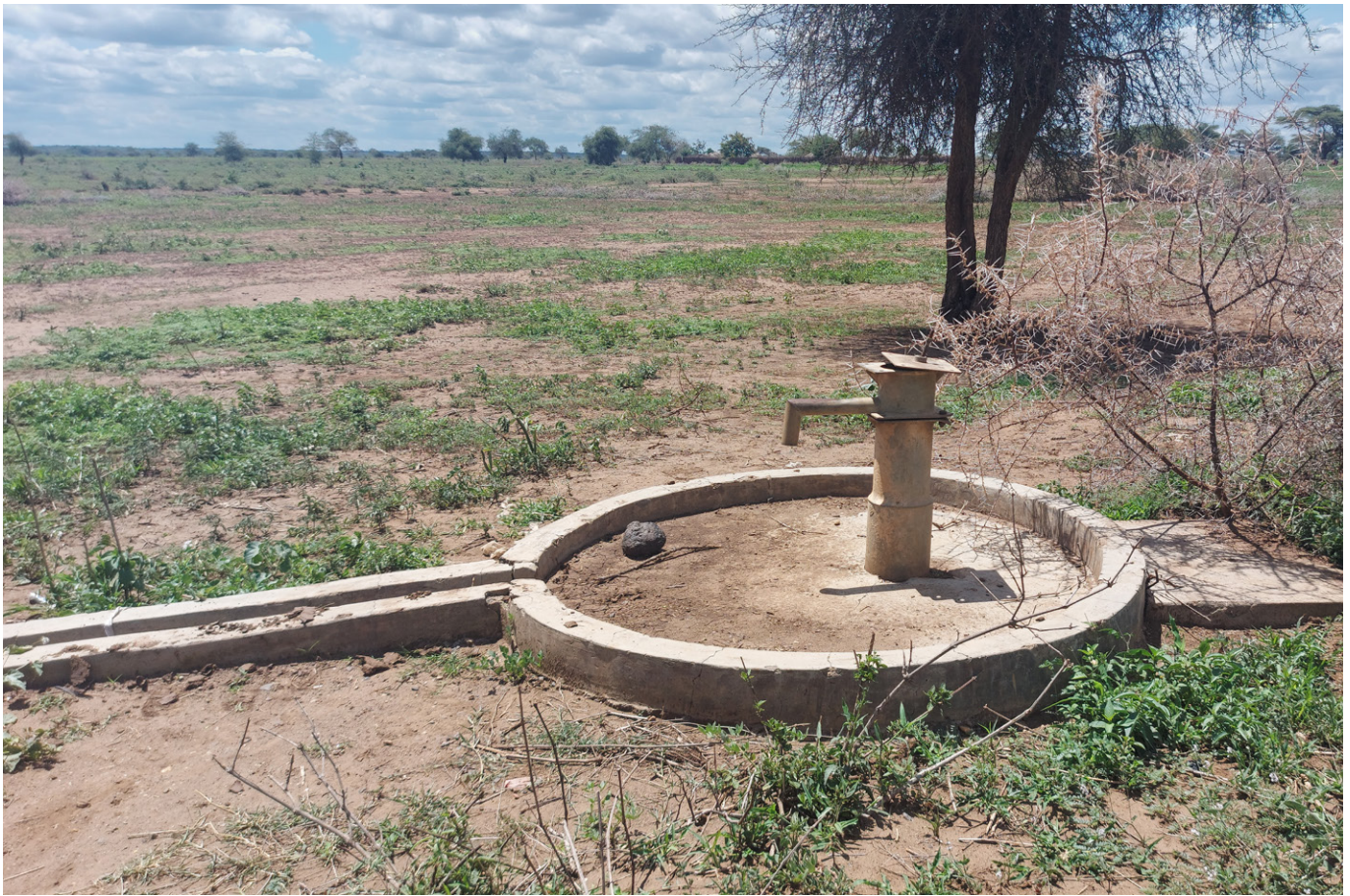
Figure 3.16 Borehole, Lokale, Moroto.
