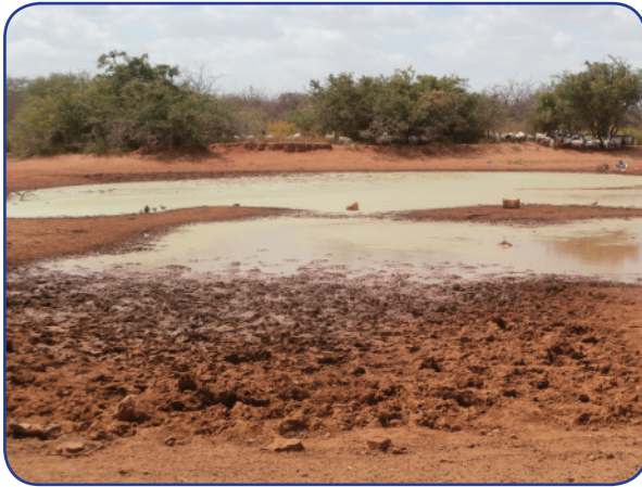
Degraded bank and contaminated water from livestock directly accessing the nearby-unimproved Harr Bibi water pan
